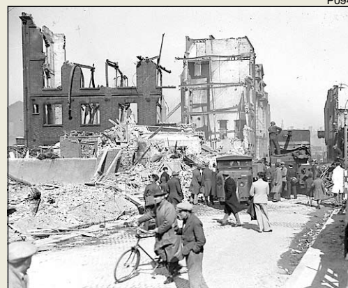
Devastation: Westwick Street in ruins.
